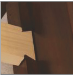
Bed Slats are Dovetailed into the Bed Rails
